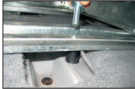
2. Seat bracket assembly removed and floating rib being attached to floor.
