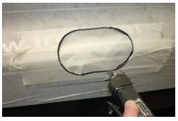
7. Drill mounting holes to 16mm.
