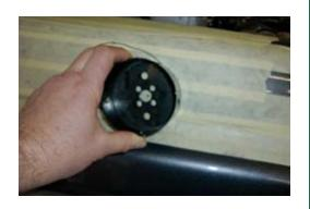
6. Drill all mounting holes to 16mm.
